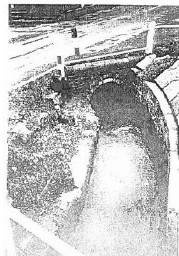
Fig 12: Headwall on downstream side of Culvert 1.
