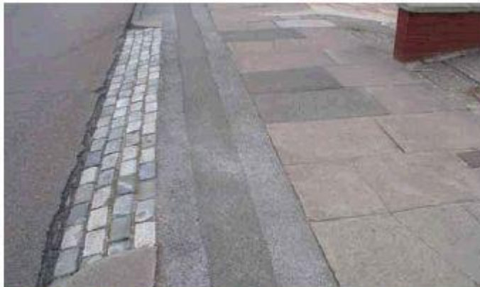
Fig 12 Design in Dunstable shows how access to driveways can be provided whilst maintaining a clear level usable width for pedestrians.
