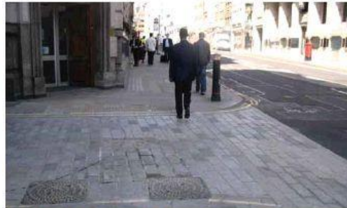
Fig 13 A raised footway extension gives disabled people and other pedestrians the most comfortable and convenient crossing point at side road junctions.
