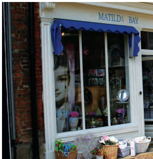
Fig 9.21 Pilaster are an important part of the shopfront and often 'contain' the fascia at both ends (Woburn)
