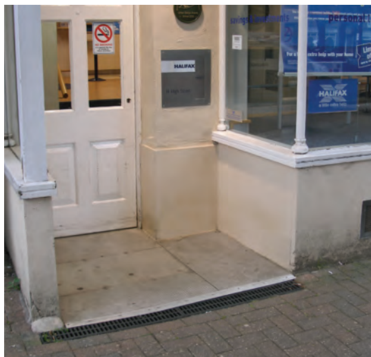
Fig 9.25 Steps removed and pavement raised to create a flush threshold to aid access. Leighton Buzzard.
