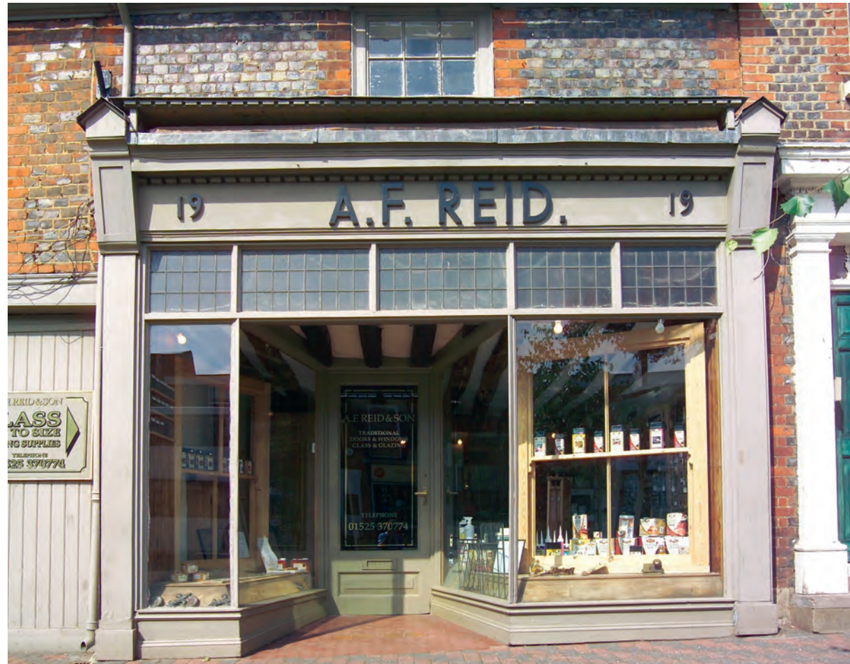
Fig 9.24 An historic shopfront skillfully repaired and conserved to create a flush threshold to aid access High Street, Leighton Buzzard.
