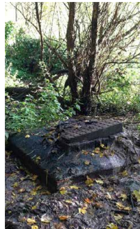
This image of a sewer overflow is the result of overstressed water infrastructure. One advantage of SuDS is their ability to remove surface water runoff from the sewer system, improving its capacity for managing wastewater.
