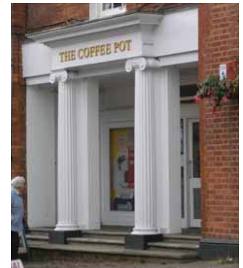
Fig 09 Integration of appropriate lettering and recessed shopfront with a classical frontage
