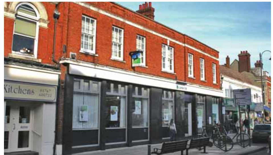
Fig 04 Biggleswade; An unbroken fascia can have a detrimental impact on the host building and is visually disruptive in the streetscene
