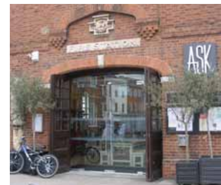
Fig 10a Sensitive retention of original openings and features and well considered location of logo. Leighton Buzzard.
