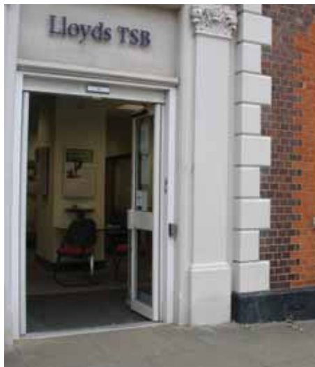
Fig 14 Pavement raised to create a flush threshold to aid access. Leighton Buzzard.
