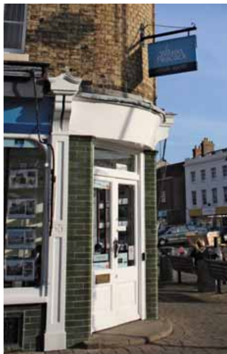
Fig 16 Signs over the highway should be a minimum of 2.1 metres (2100mm) above the highway. The sign shown is well positioned and takes maximum advantage of the architectural composition of the corner entrance to this shopfront in Biggleswade.
