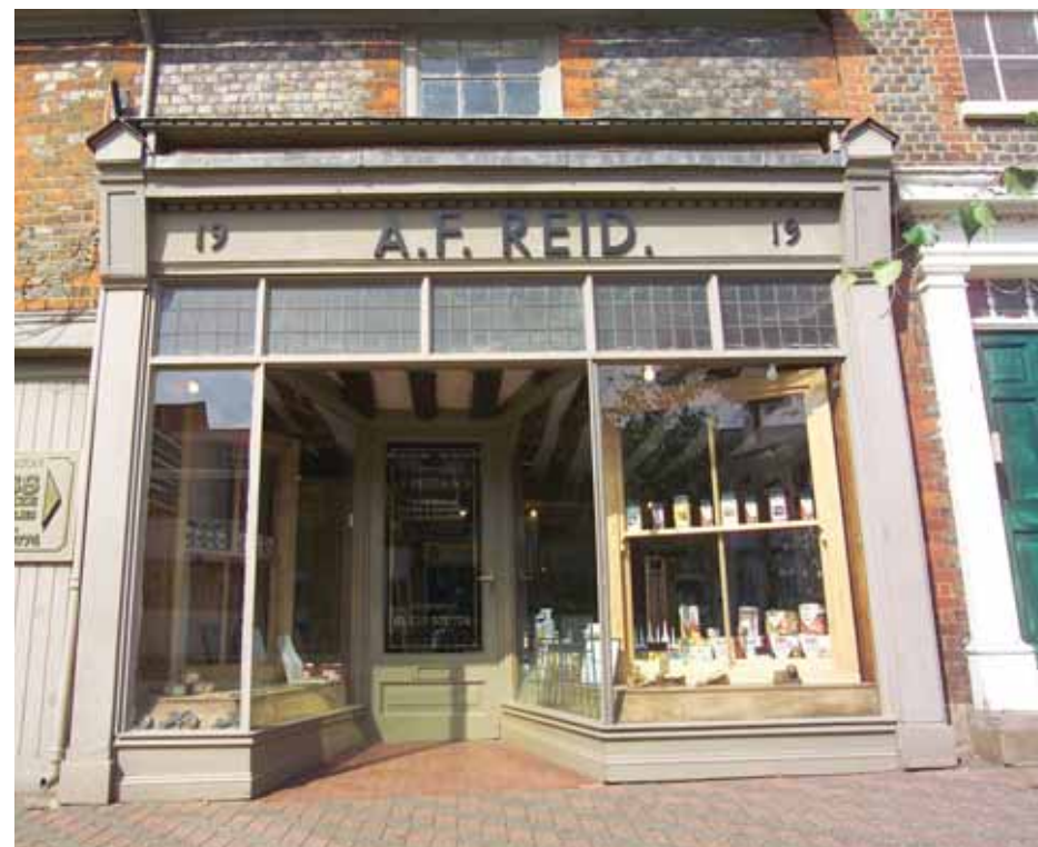
Fig 13 An historic shopfront skilfully repaired and conserved. High Street, Leighton Buzzard.
