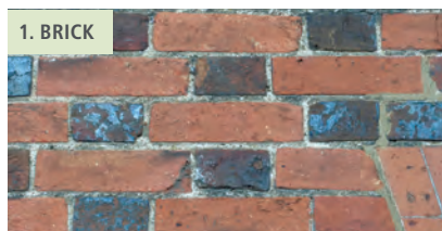
1a Red brick in Flemish bond with burnt headers
