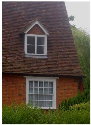
Fig 22. A small paned vertical sliding sash window with a side hung dormer casement above (The Red House, The Green)
