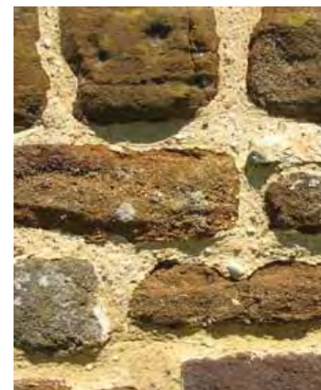
Fig 22 Ironstone repointed using lime mortar and a sharp gritty sand providing a traditional finish which will preserve the integrity of the historic stonework.
