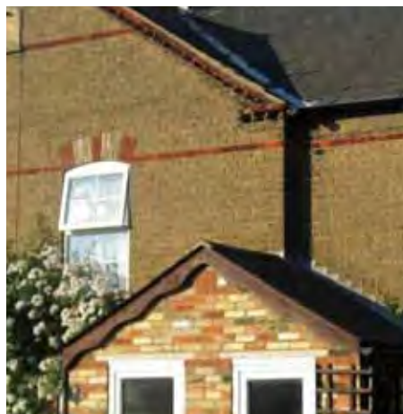
Fig 31 Poorly considered additions to traditional buildings – uPVC windows and unsympathetically designed enclosed porch. The random use of salvaged bricks of various colours is intrusive.
