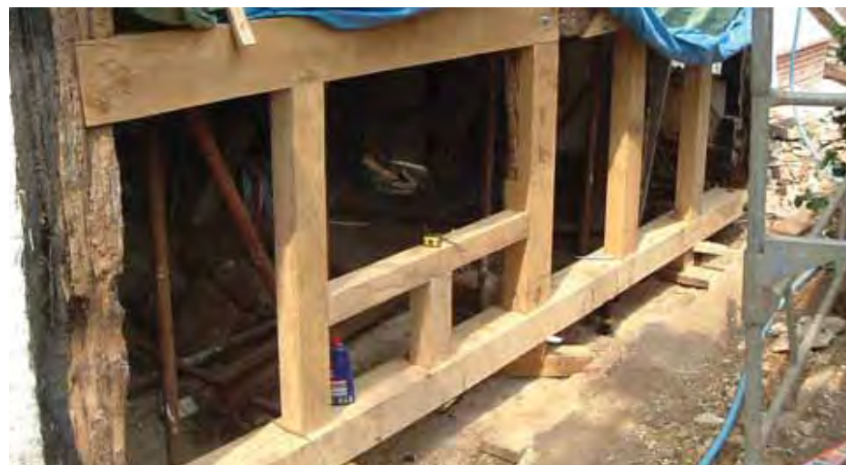
Fig 16 Example of good practice timber repair – sections of timber being spliced in retaining as much of the historic fabric as possible
