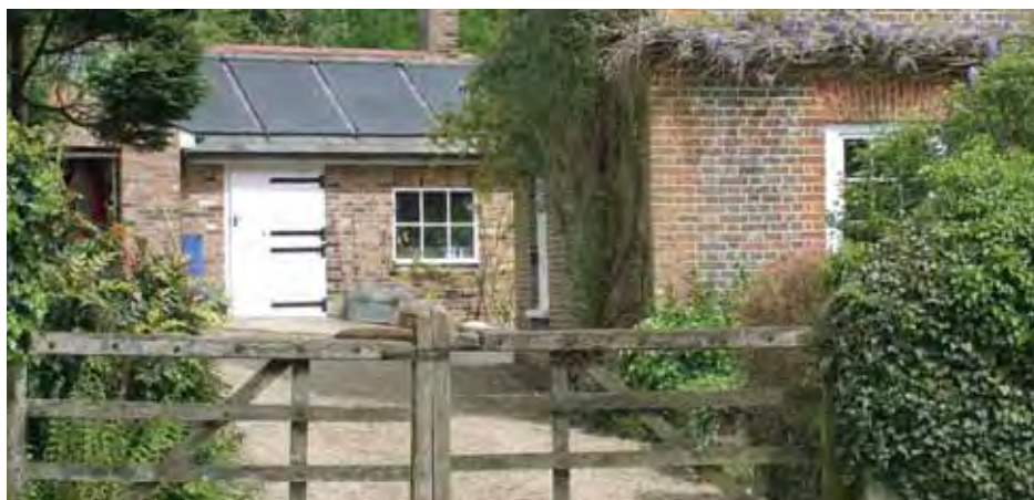
Fig 23 Photovoltaic panels located on outbuildings rather than the larger main buildings in order to reduce their impact. Kensworth, Church End.
