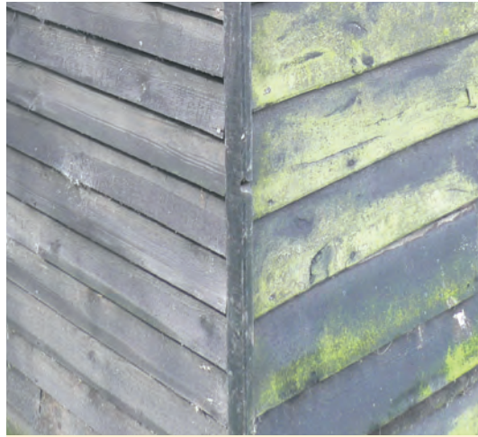
Fig 3.36 Barn at Barton le Clay showing different depths of weatherboarding
