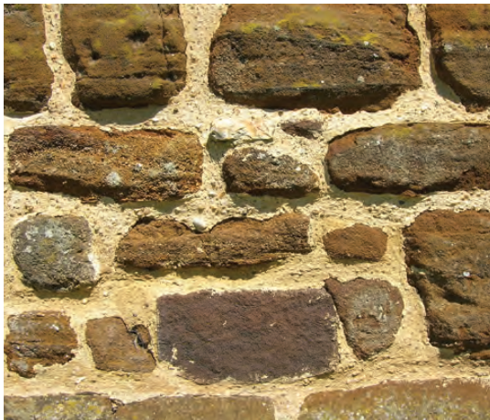
Fig 3.35 Ironstone repointed using lime mortar and a sharp gritty sand providing a traditional finish which will preserve the integrity of the historic stonework
