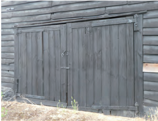
Fig 3.48 New openings should be kept to a minimum and cart openings and doors such as those at Crawley Hall Barns, Husborne Crawley should be retained as part of a conversion scheme.
