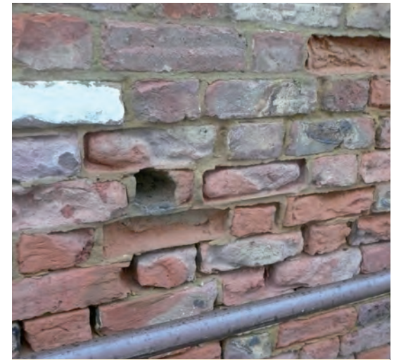
Fig 3.39 The damaging effects of cement pointing
