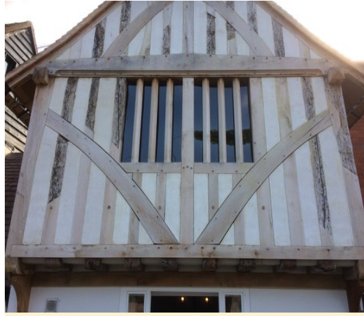
Fig 3.37 A tidy and painstaking example of historic timber frame reconstruction where extensive frame component replacement was required
