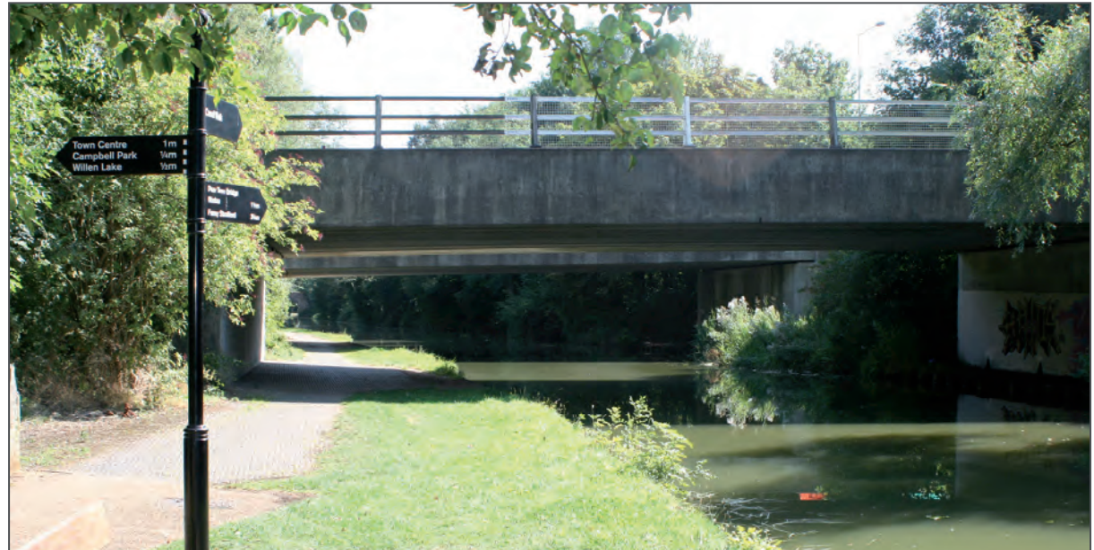
Fig 2.27 Underpass allows not only aquatic life to pass in the canal, but also provides a means of dry habitat connectivity
