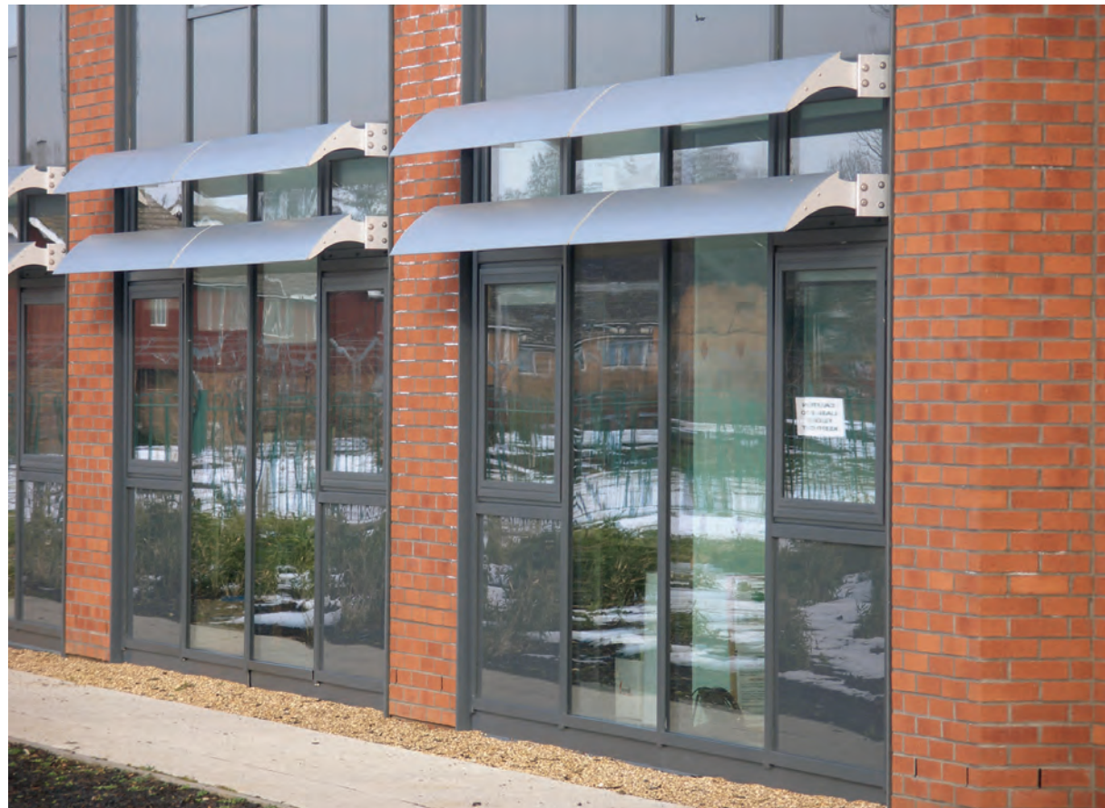
Fig 8.12 External louvers on a western elevation. These are effective at most times of the year, although low winter sun is a challenge for the design of any shading device.
