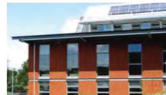
Fig 8.02 Roof profile integrating photovoltaics and window shading on south facing elevation.
