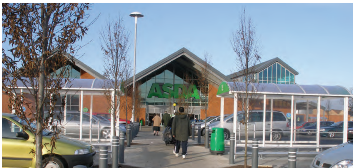
Fig 8.03 Large span foodstore with structural bays expressed and south facing walls recessed to create shading. Note also large glazed areas allowing daylighting and creating an active frontage.
