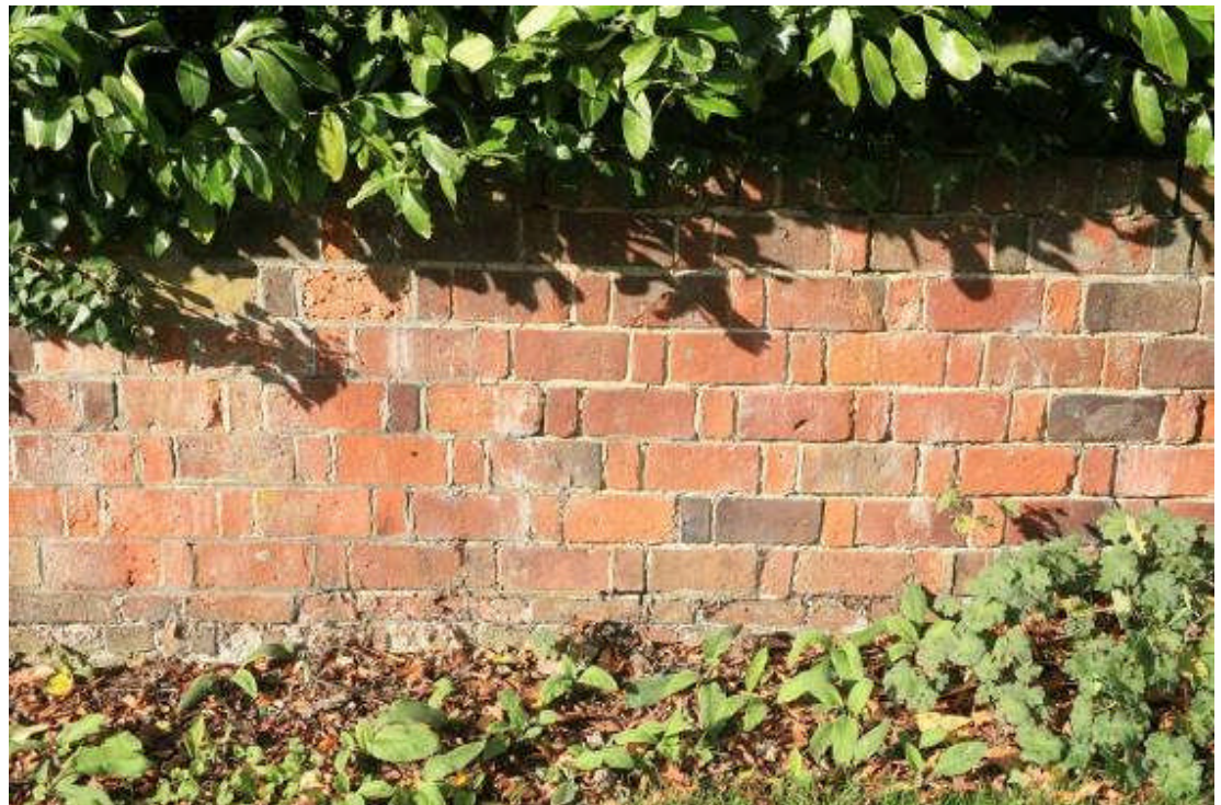
Brick boundary wall in distinctive Rat-trap bond, Manor Farmhouse
