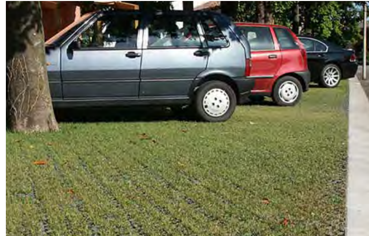
FIG. 6.7 Re-inforced grass car parking for attenuation
