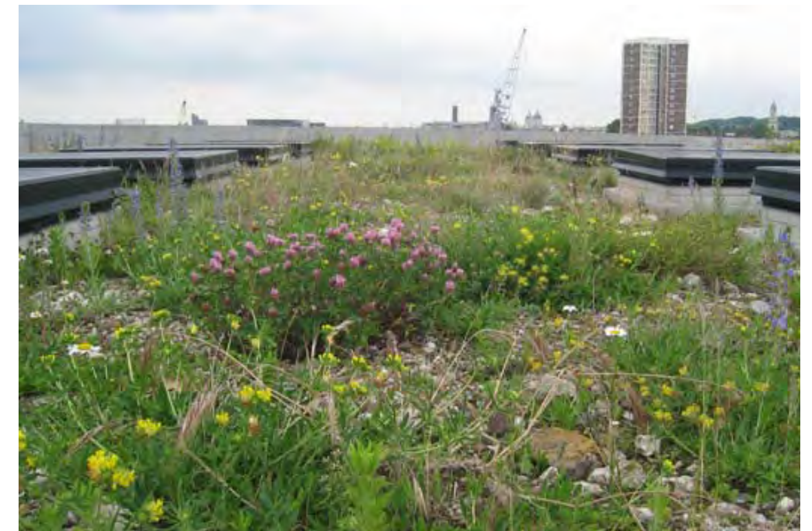
FIG. 6.11 A green / brown roof for habitat and attenuation
