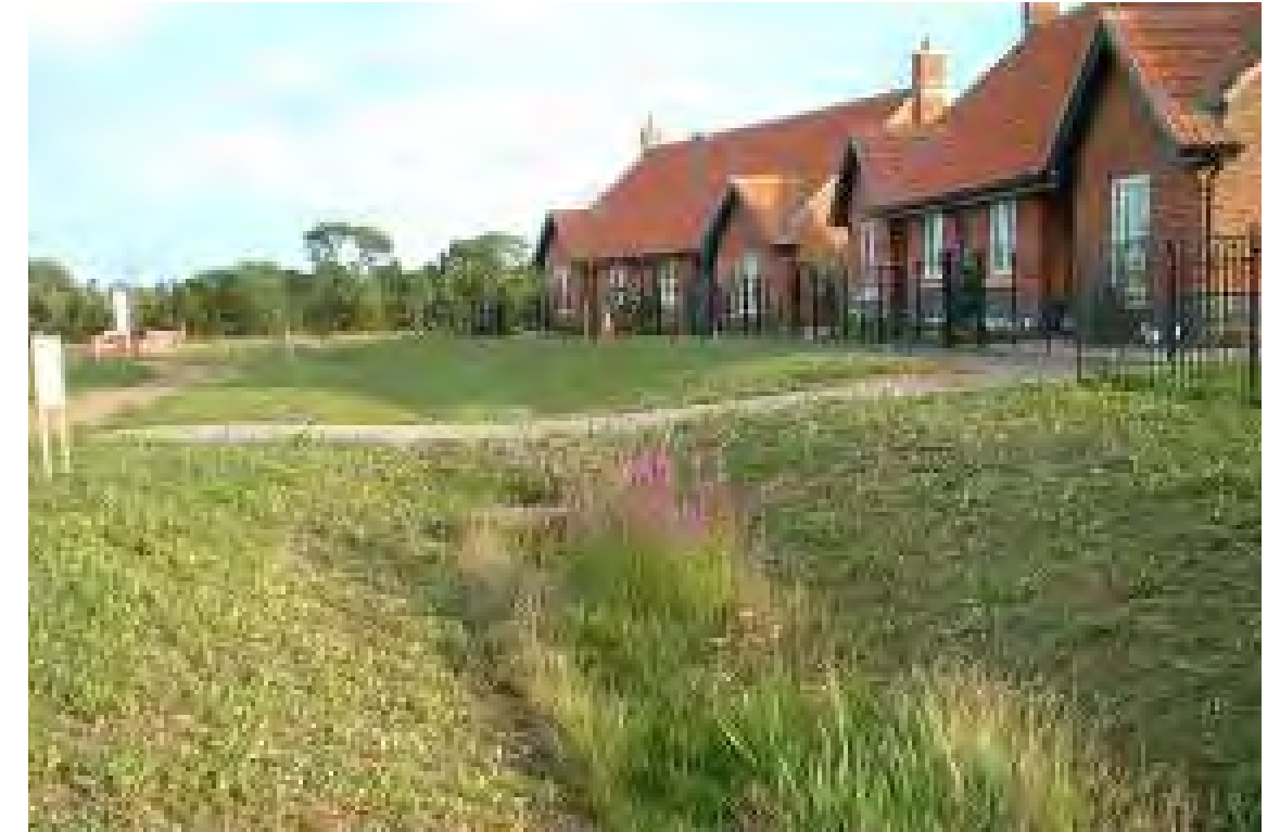
FIG. 6.10 A swale for rainwater attenuation
