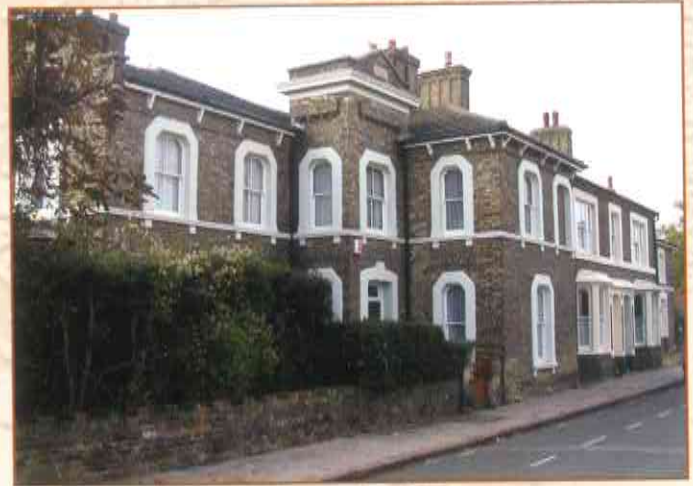
Entrance tower to no.12 Station Road
