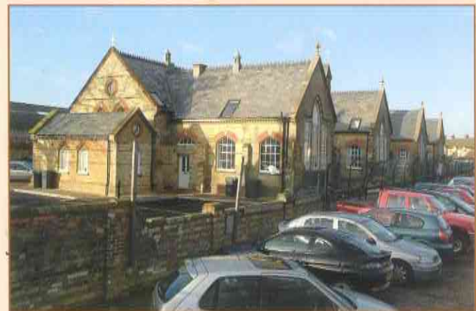
Claremont Court (residential conversion of former Victorian School)
