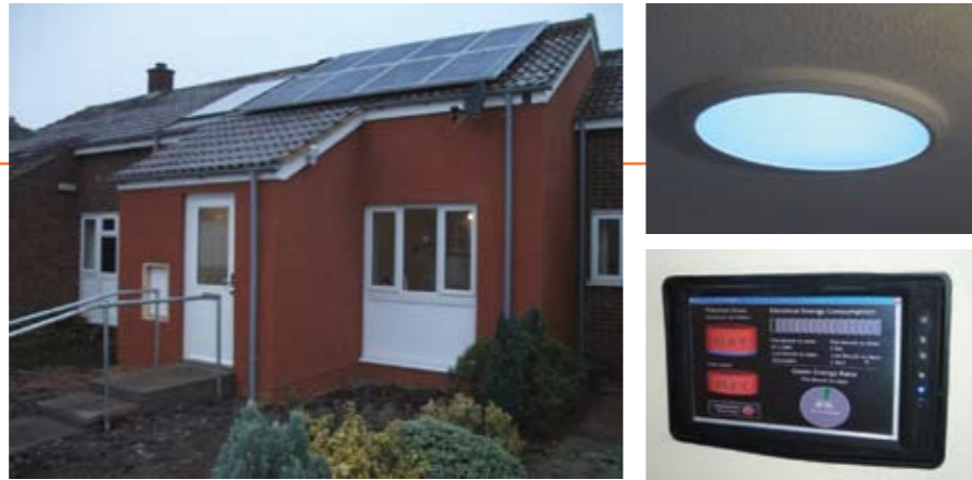
The eco-makeover included solar panels, sun pipes and energy meters
